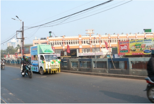
Saldah Station Flyover
